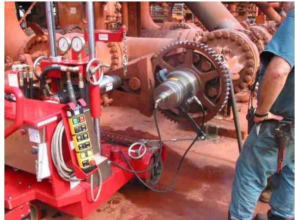
The valve grinding unit undergoing site trials.
